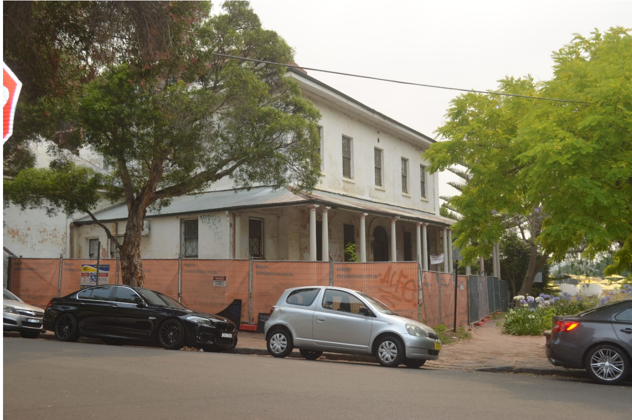
corner of Buckingham Street and Bedford street - looking west
