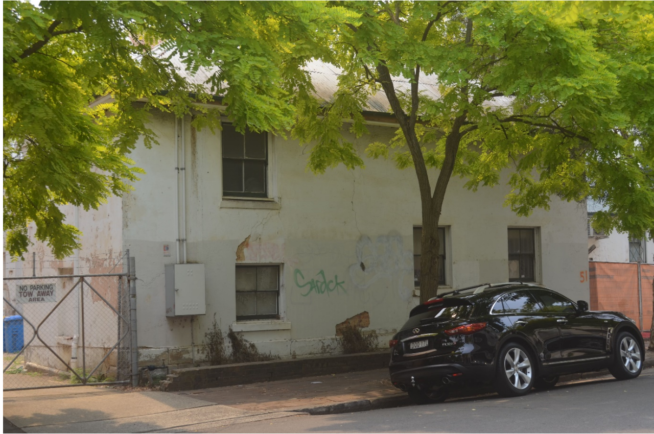
side/rear of site - Buckingham Street
